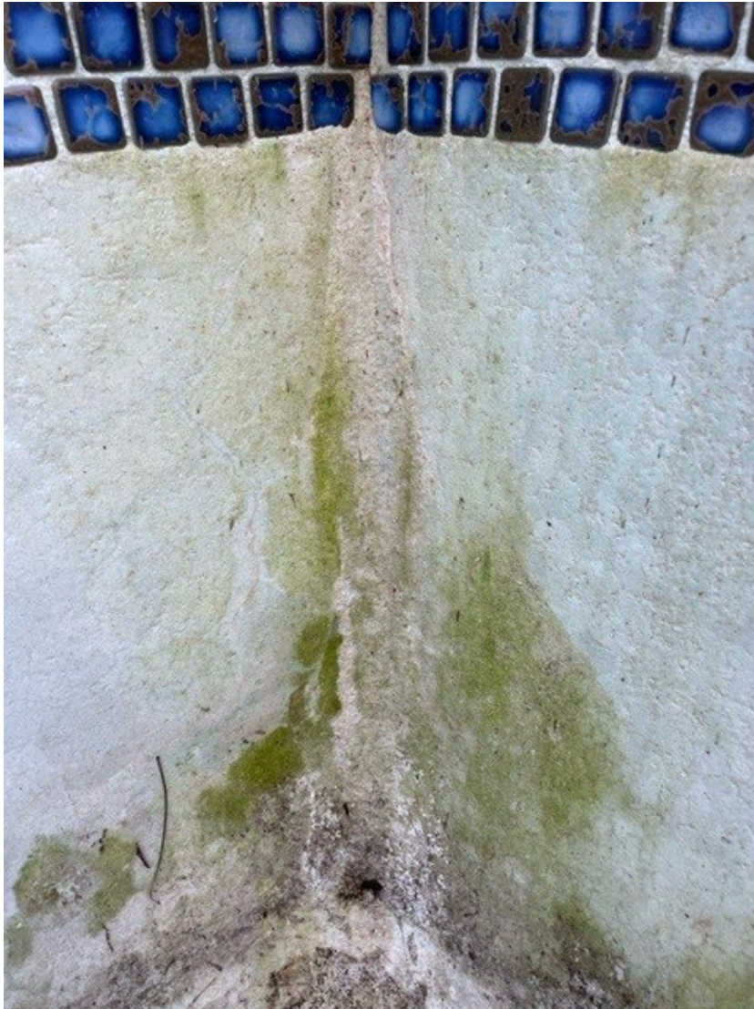
Additional Pool Photos: Shallow end previous repair
