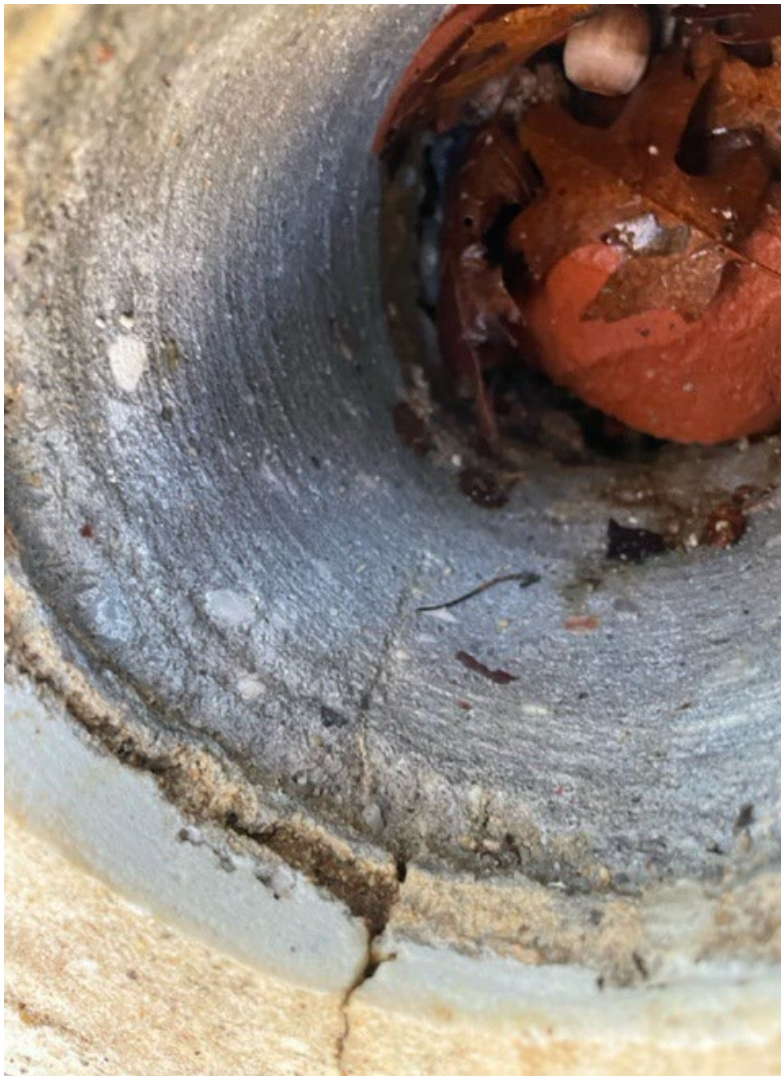
Additional Core Through Crack in Pool Floor
